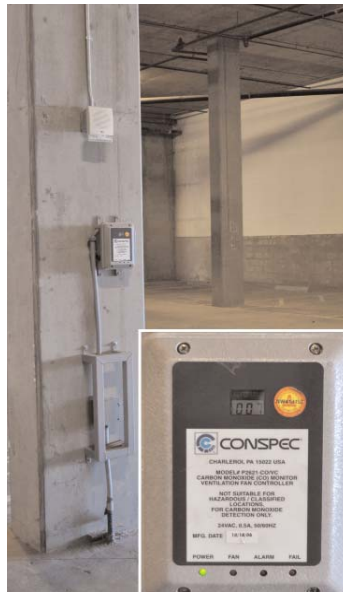
A monoxide ventilation fan controller unit installed in an underground parking facility in Los Angeles, CA demonstrates a typical installation and the recommended installation height as shown in the "breathing zone" to ensure personal safety.
